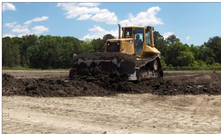
Ponds were drained (above), filled with clean soil, and the contaminated soils and sediments mixed with concrete and additives. The mix was used as a sub-cap over the site (below).
