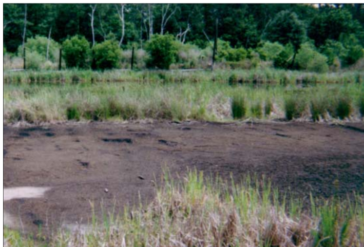
Ponds were drained (above), filled with clean soil, and the contaminated soils and sediments mixed with concrete and additives. The mix was used as a sub-cap over the site (below).
