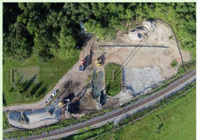
Brunswick Wood Preserving Site: Treated soil stockpile relocation
