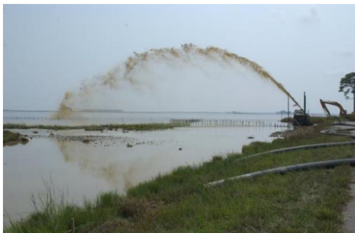
Example of thin layer being implemented on the marsh.
