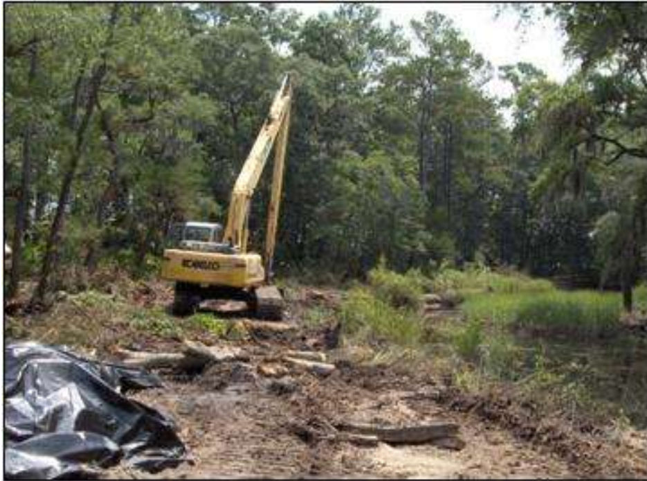
Contaminated sediments are being removed from Burnett Creek during periods of low tide.
