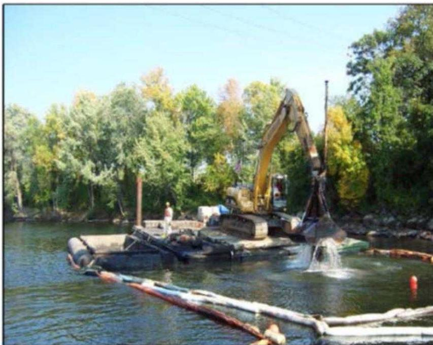
**Capping** – Cover the contaminated sediment with layers of sand, silt, gravel and rock designed to contain and isolate the contamination. This is also called “containment.”
